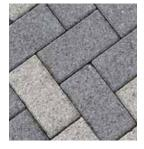
**Pavers:** Paver driveways offer a high-end look with many design possibilities. Made from materials like brick or stone, they are durable and can be easily repaired by replacing individual pieces. However, pavers tend to be more expensive and laborintensive to install.
